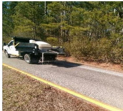
Applying brine solution to the road
