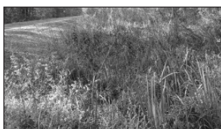
A wide, shallow drainage area can reduce erosion and control sediments. Photo by Bruce Nichols, NRCS
