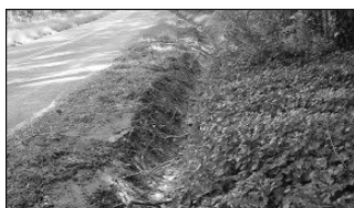
Bare soil in this ditch will erode and contribute to pollution downstream. Photo by Bruce Nichols, NRCS
